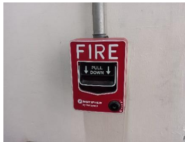
Fire Alarm Manual Station
